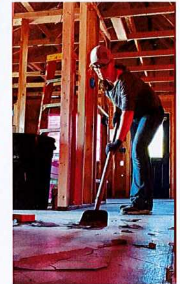
Brittany Satterwhite prepping for new flooring in Ely
