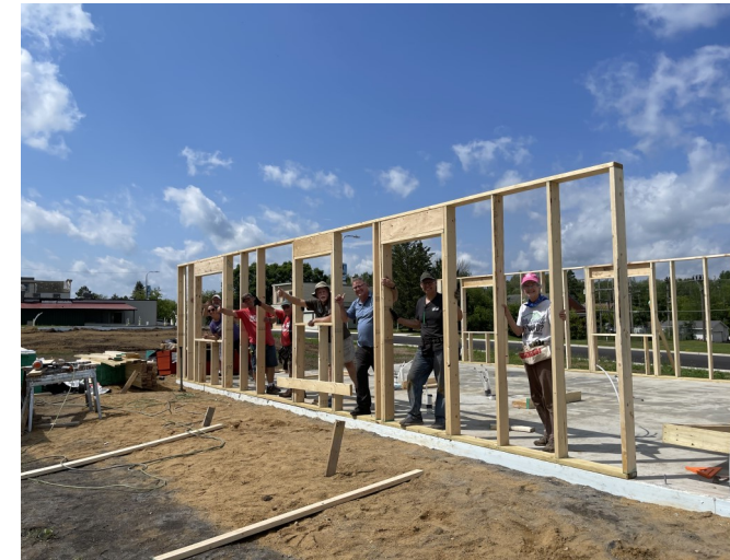
Wall Raising in Buhl with Care-a-Vanners
