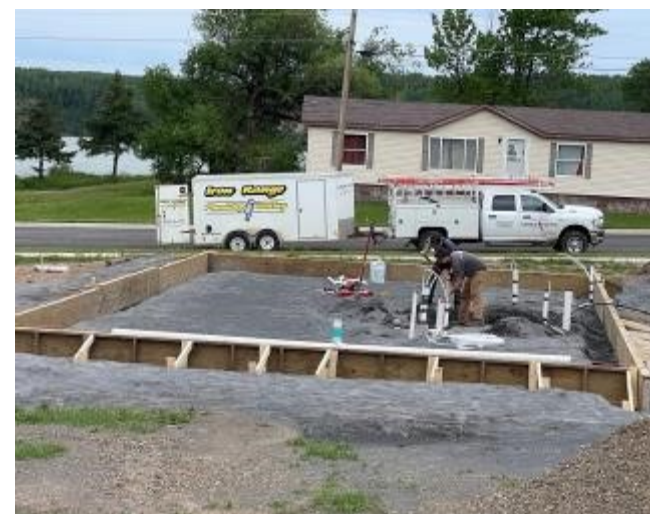
Plumbing install in Buhl with Iron Range Plumbing and Heating
