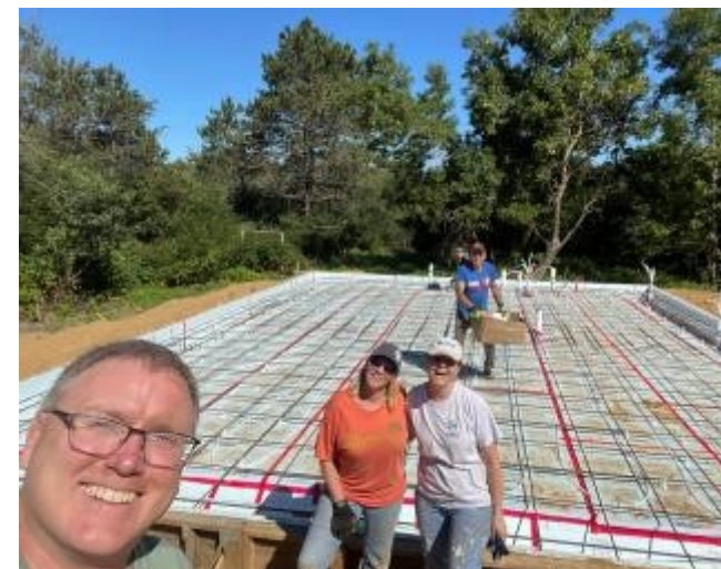
Foundation work in Hibbing with 3D Concrete and Staff
