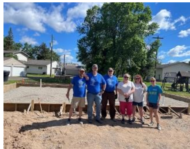
Foundation work in Virginia with Blue Cross Blue Shield
