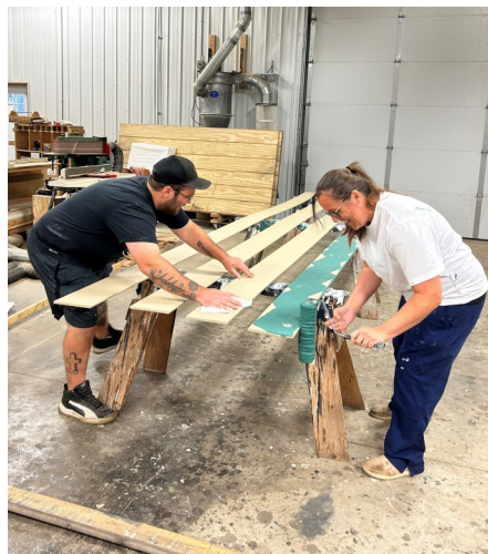
Homebuilders Nick and Cree painting their exterior siding.
